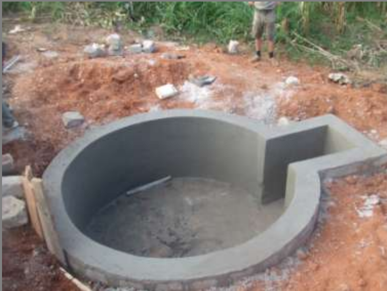
Biogas Digester – Construction Process
